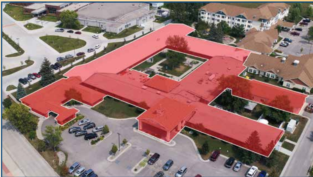
The areas of the building indicated in red experienced significant damage from the fire and will be rebuilt.
